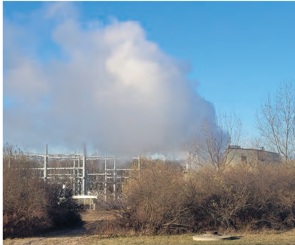
SMOKE STACKS: The view from directly outside the RIRRC headquarters on Shun Pike shows a beehive of activity. RIRRC runs the Ocean State's lone operating Central Landfill. RIRRC oversees Rhode Island's Materials Recycling Facility, Leaf and Yard Compost, and Eco-Depot. (Sun Rise photos by Rory Schuler)
